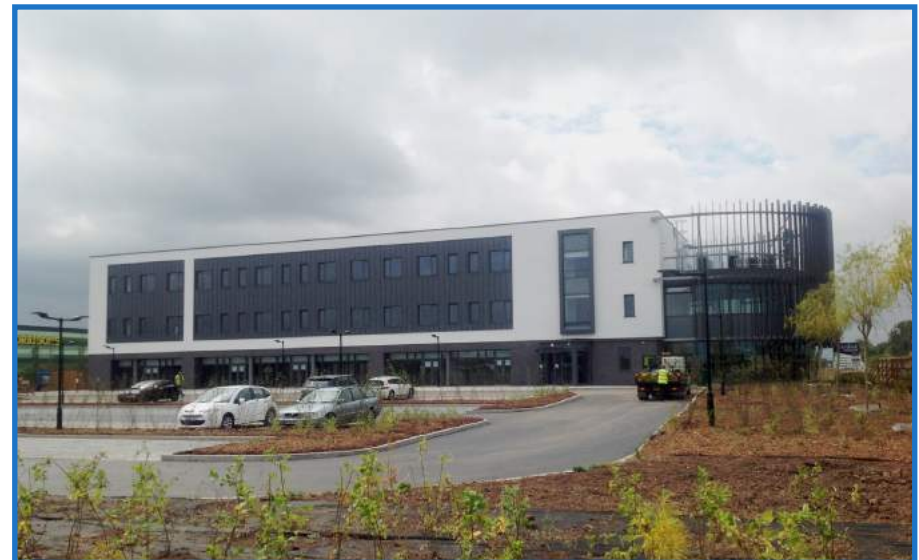
Somerset Energy Innovation Centre
